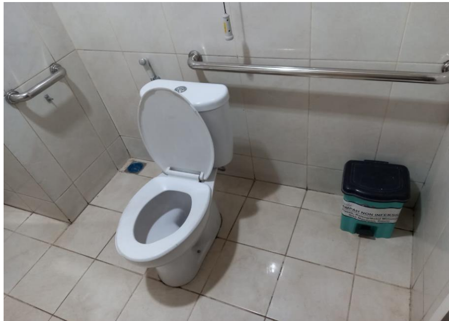
TOILET DISABLE GARUDA LANTAI 1
